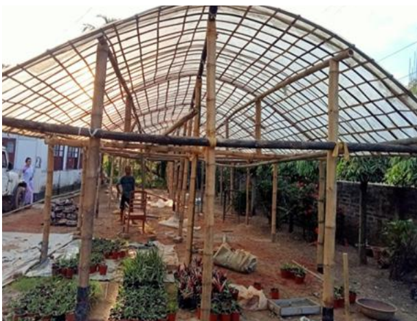
Low cost vegetable nursery constructed using locally available bamboo under construction
