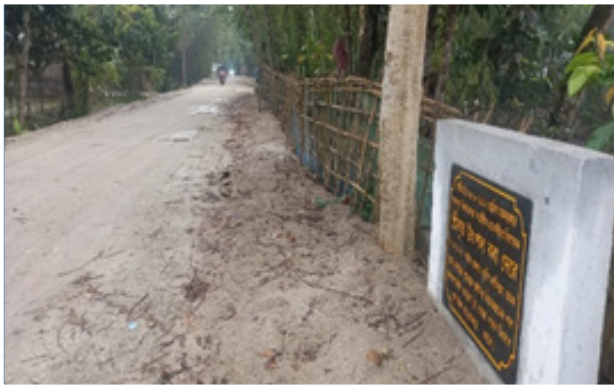
Road construction is underway
