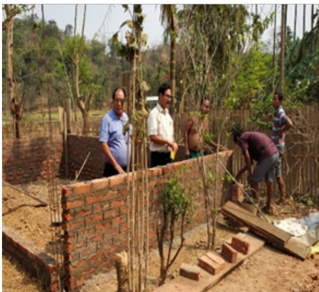
Construction of eri rearing house in progress
