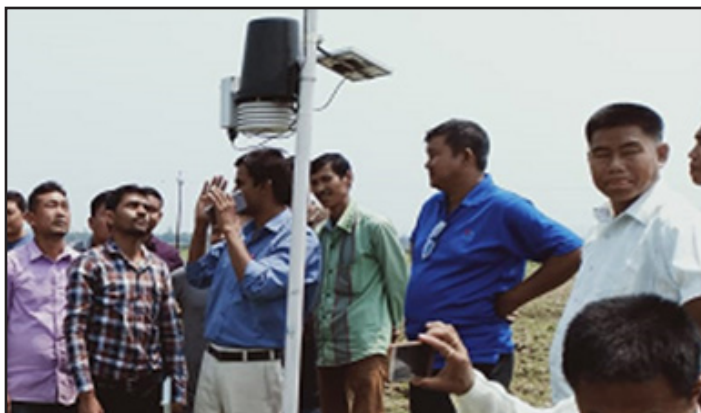
Weather stations installed in the villages
